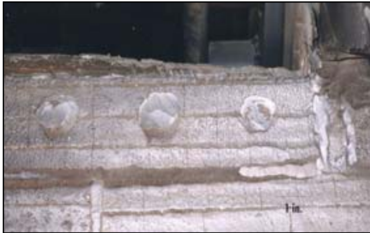
Vanadium Carbide Weld Overlay After 14 Months (19 mm ( \frac{3}{4} " ) eroded from leading edge)
