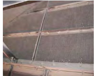
Conforma Clad screens after 9 months.
